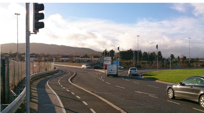
Figure 8: Looking South, the existing narrow two way cycle track
