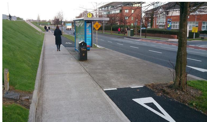
Figure 11: Unfinished cycle track where Bus Stop remains in the way of cycling. Picture taken in January 2014.
